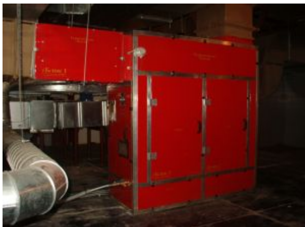
Picture 2 - «Gasconvector «Yatagan» on the object (presentation of the company «Ecopromika»)
