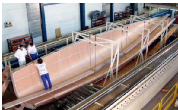
Picture 1 – Preparation of the mold surface for further reinforcement layer applying (presentation of the company «Tehno express»)
